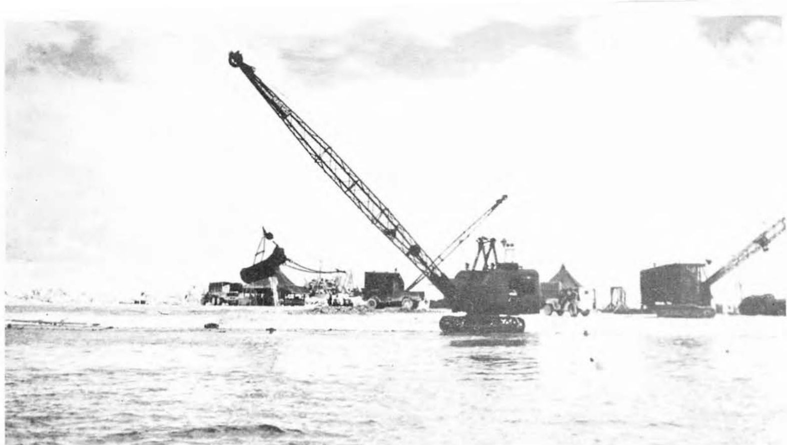
DREDGING ORANGE BEACH CHANNEL
